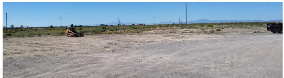
Clearing and leveling plant site
