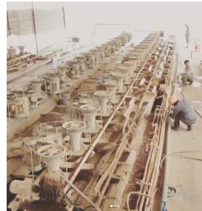
Fluorspar flotation plant
