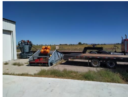
Assembling plant components
